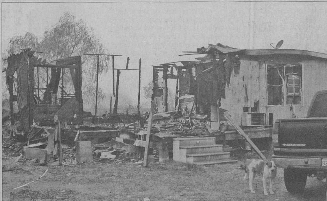
Pictured above is what remains of the Jones Residence at 4878 FM 102 South. A fire in the early hours of Monday, December 7 destroyed the home and claimed the life of Troy Richardson, a seventh grader at Rice Junior High. Richardson lived in the home with grandparents Andrew and Deborah Richardson. No cause for the fire had been established as of press time.
